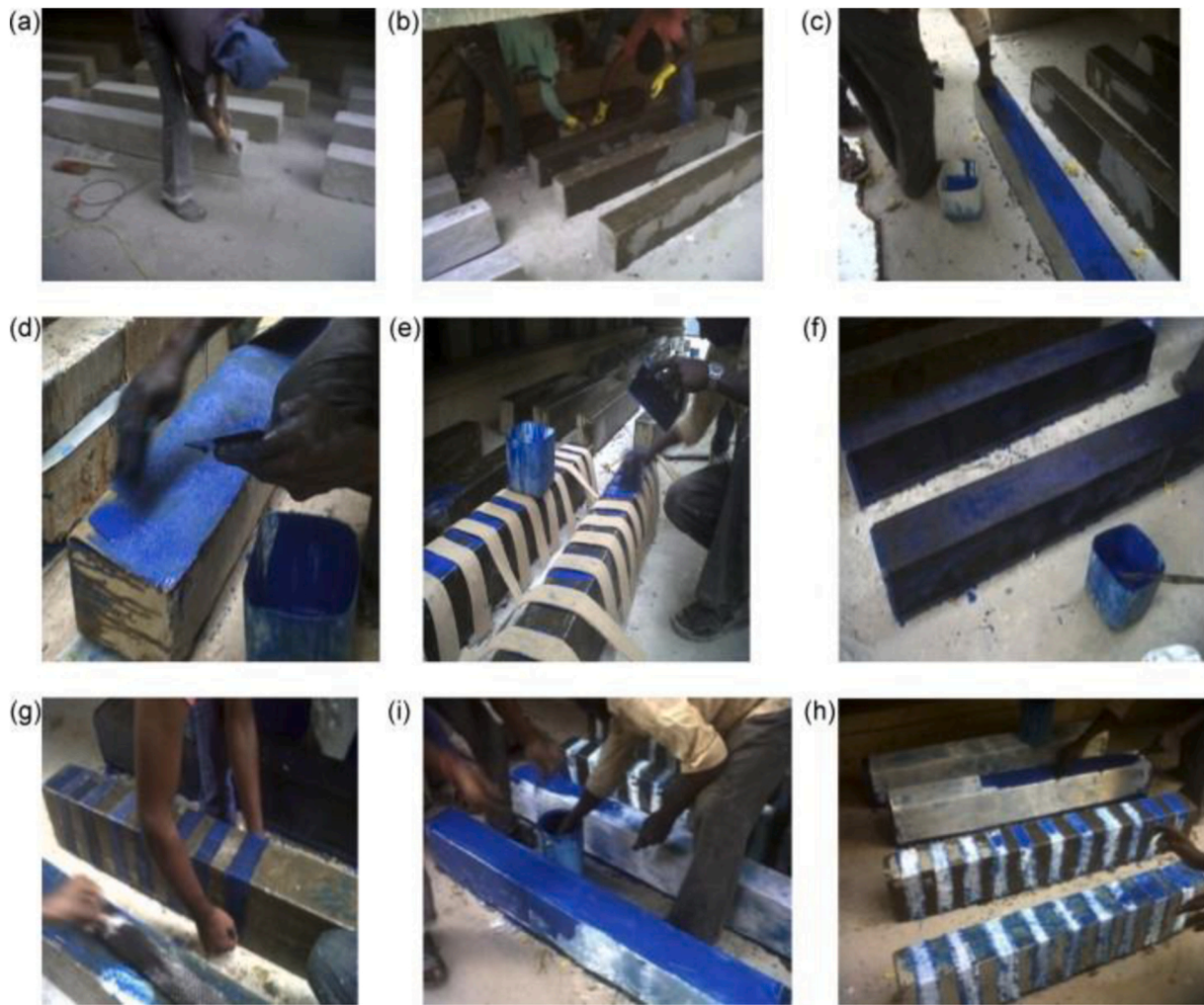
Fig. 24. Application case of NF in reinforced concrete beams, reproduced under license number 5491290642595 from [167].
