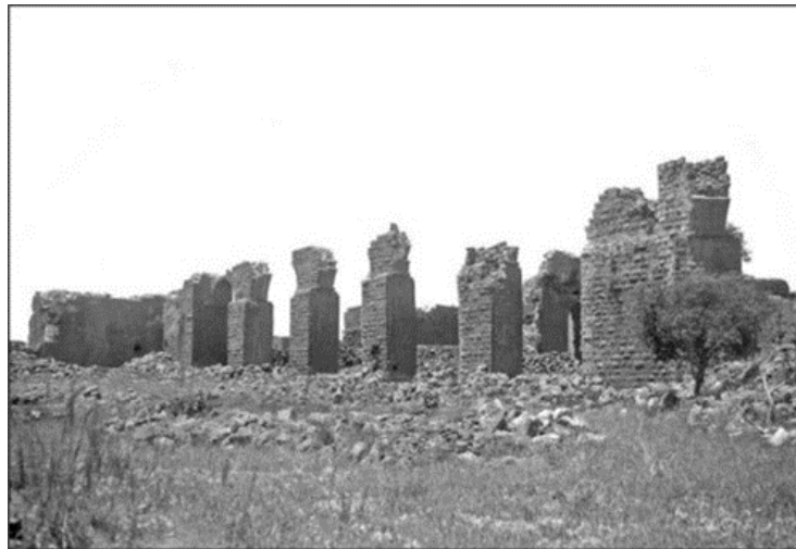
Fig.8 The Roman aqueduct in Shahba (Brünnow 1909)
